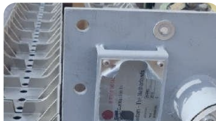
Duct burner replacement
