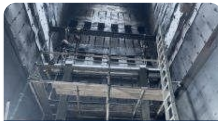
Boiler header replacement
