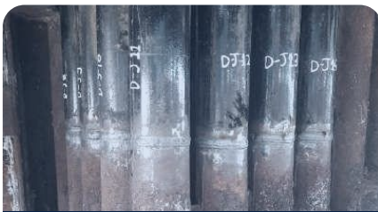
Boiler tube bundle replacement
